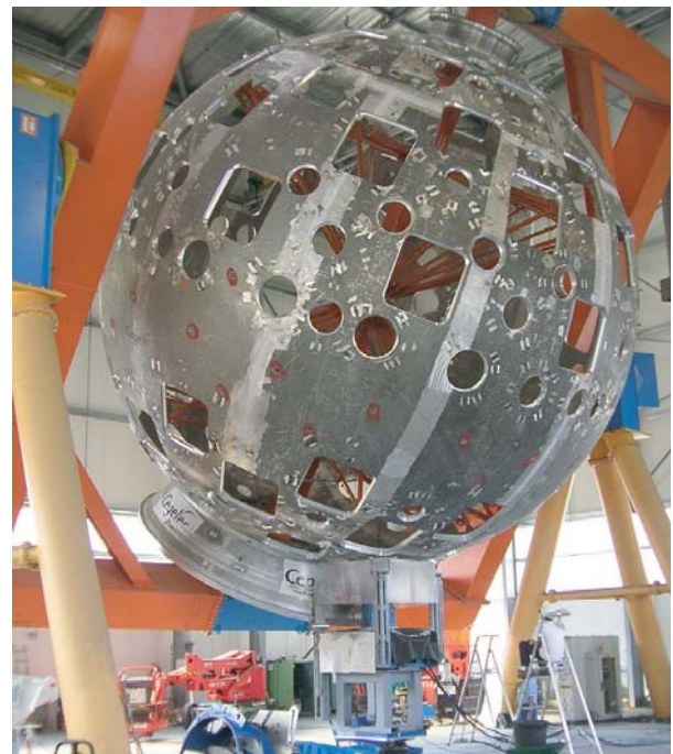
Fig. 13. (Color online) Target chamber under construction.
