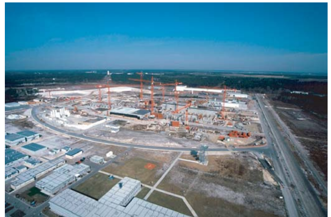
Fig. 12. (Color online) General view of the construction site.
